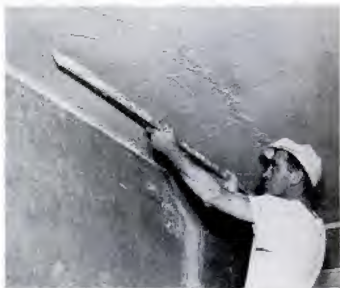
Plasterer uses rod (straightedge) to level surface and remove excess. Final leveling is done with darby (long float) which also produces roughened surface
